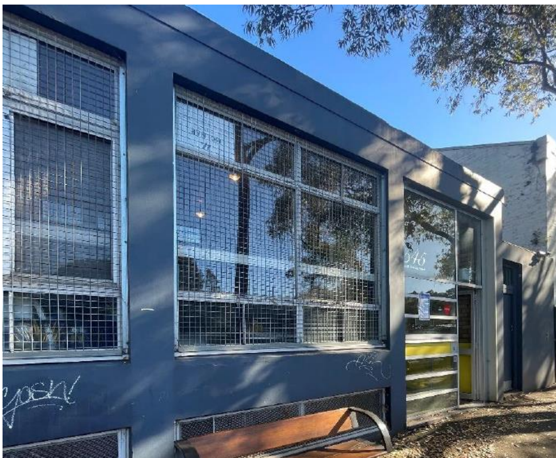
Figure 2: Subject site and existing entrance from South Dowling Street
