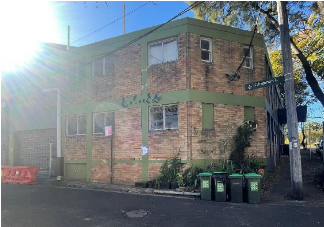
Figure 4: Subject site viewed from the corner of Chapman Lane and Phelps Street
