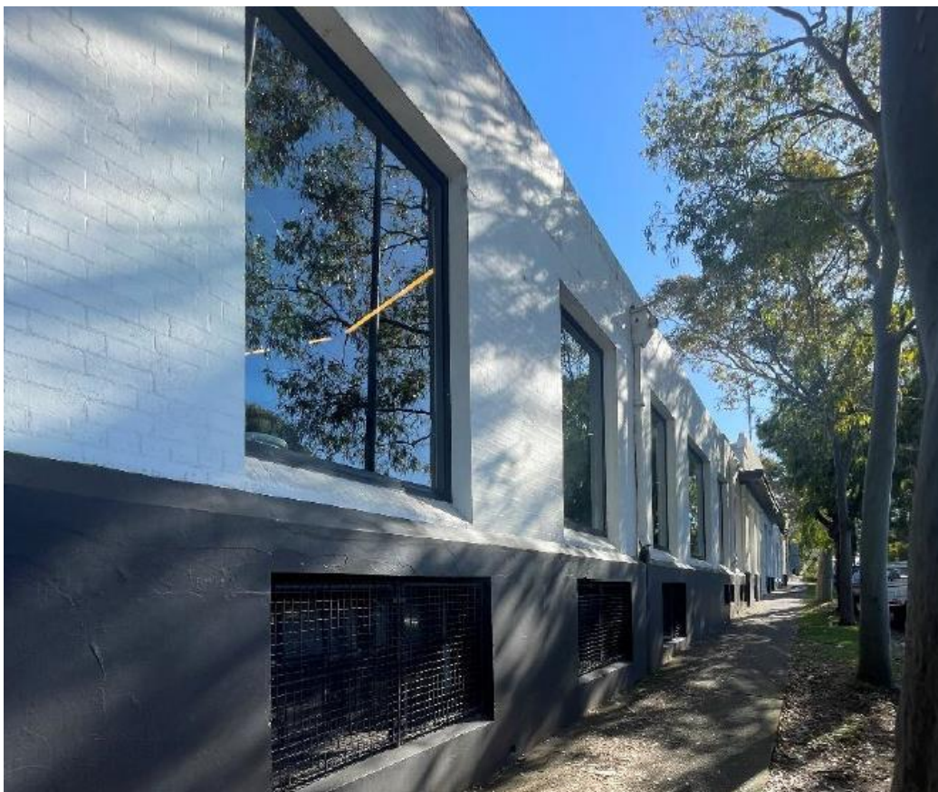
Figure 6: View of 515-543 South Dowling Street (immediately north of the subject site)
